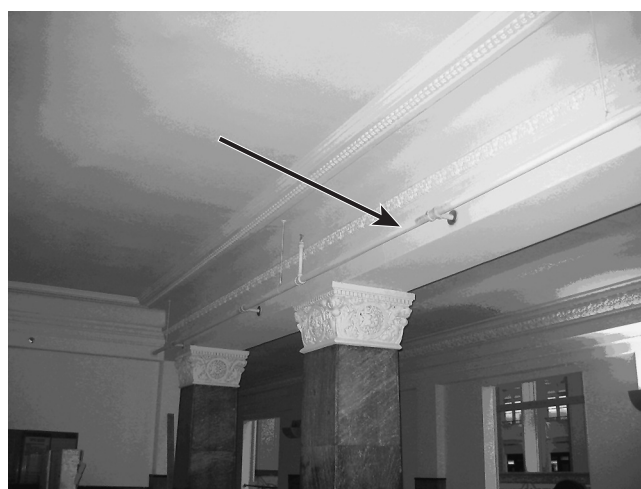
FIGURE F.3(e) Sprinkler Piping Out of Normal Sight.
