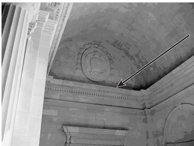
FIGURE F.3(c) Exposed Sprinkler Pipe.
