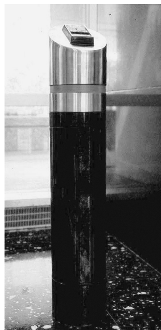
FIGURE F4(d) Bollard-Mounted Fire Alarm Station.
