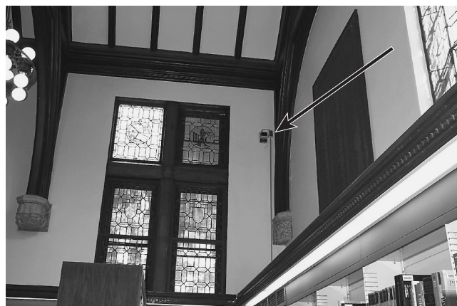
FIGURE F4(c) Linear Beam Smoke Detector.
