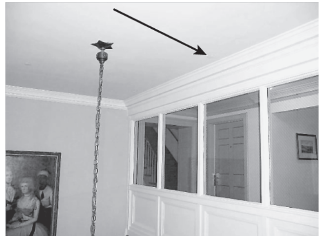
FIGURE F.3(a) Sprinklers to Maintain Glass Cooling.
