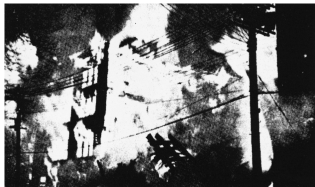
Figure 2-10.1(a) The 2-story vault [see Figure 2-10.1(b)] was in this sprinklered 4-story brick, plank-on-timber hardware factory in Syracuse, NY. The $977,000 fire was detected by the security guard. After this fire of suspicious origin was extinguished, sprinkler valves were found shut off.
