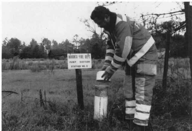
Figure B-5.6(a) A dry fire hydrant innovation has eliminated the top 90-degree or 45-degree elbow on each hydrant. (Photo by Nahunta Volunteer Fire Department, NC)
