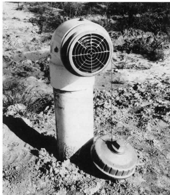
Figure B-5.1(a) Dry hydrant.
