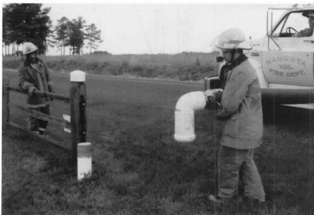
Figure B-5.6(b) Hard suction hose is connected to the pumper. The driver maneuvers the truck as the fire fighter walks the suction end of the hose to the dry fire hydrant. An "O" ring in the plastic "L" provides a right fit and allows the operator to draft. This is a quick and simple method to connect the pumper to a dry fire hydrant. It is critical that a good seal be obtained with the "O" ring to prevent any air leakage, or the pump will fail to prime.
