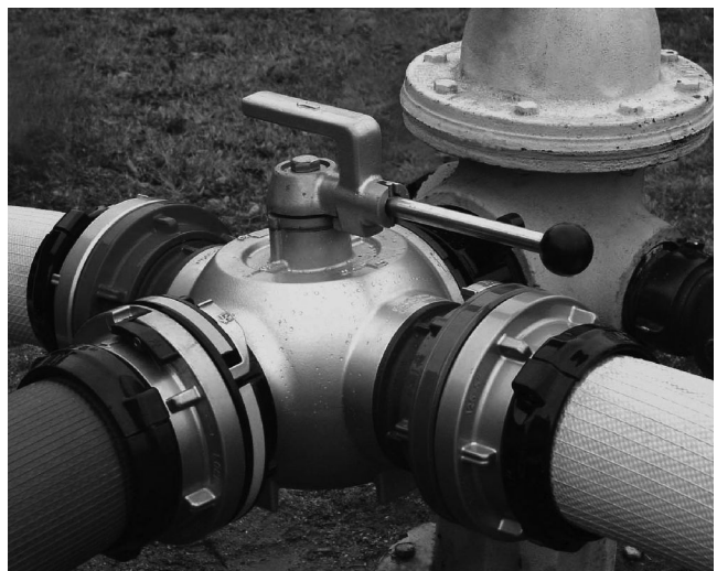
FIGURE D.5.2(b) Four-Way Hydrant Valve in Use. (Courtesy of Kocheck Co., Inc.)
