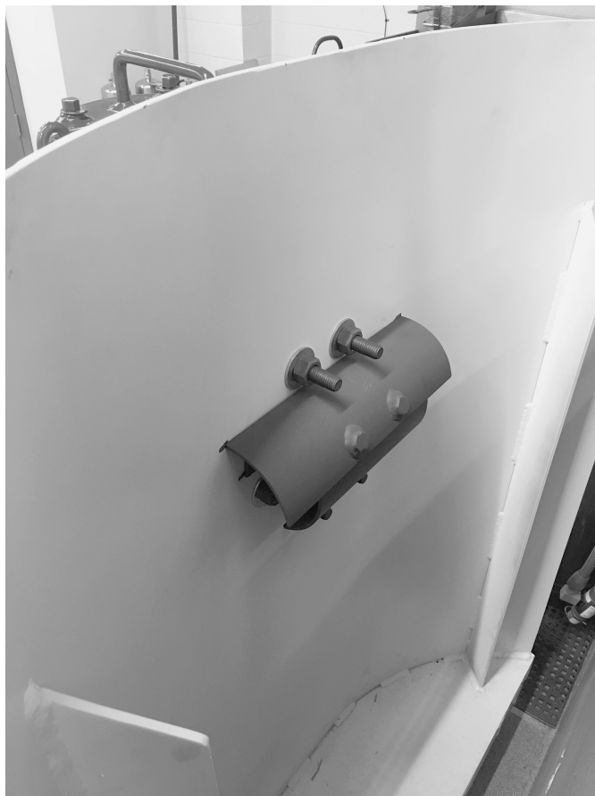
▲ FIGURE A.5.2.5.2.1(b) Foam Chamber Deflector.
