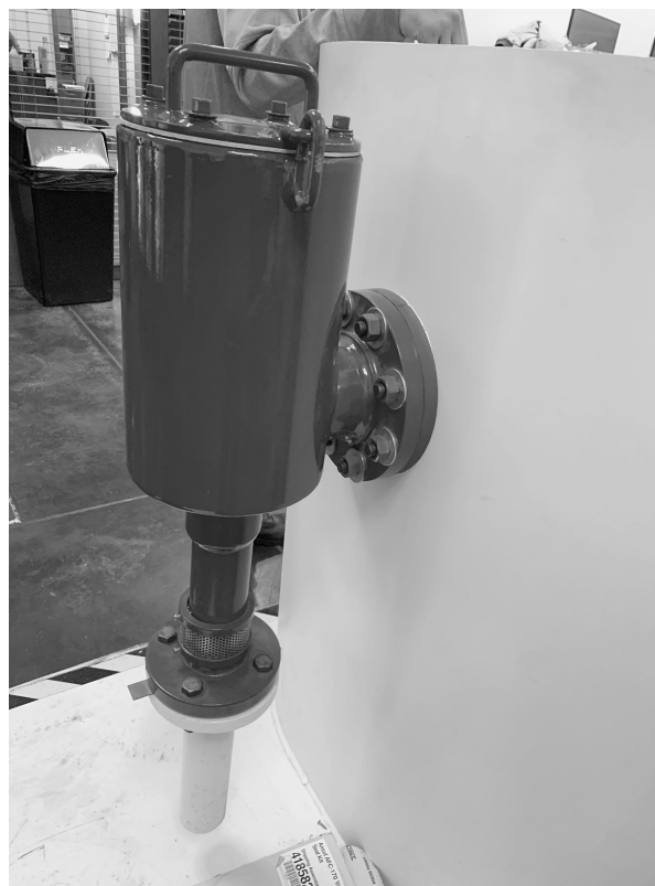
▲ FIGURE A.5.2.5.2.1(a) Foam Chamber.
