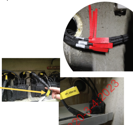
Figure B.5 – Example for field marking (cables)
