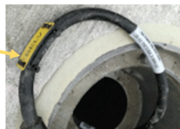
Figure B.4 – Example for field marking (inset luminaires)
