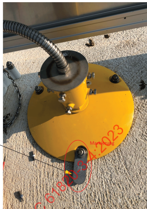
Figure B.3 – Example for field marking (elevated luminaires)
